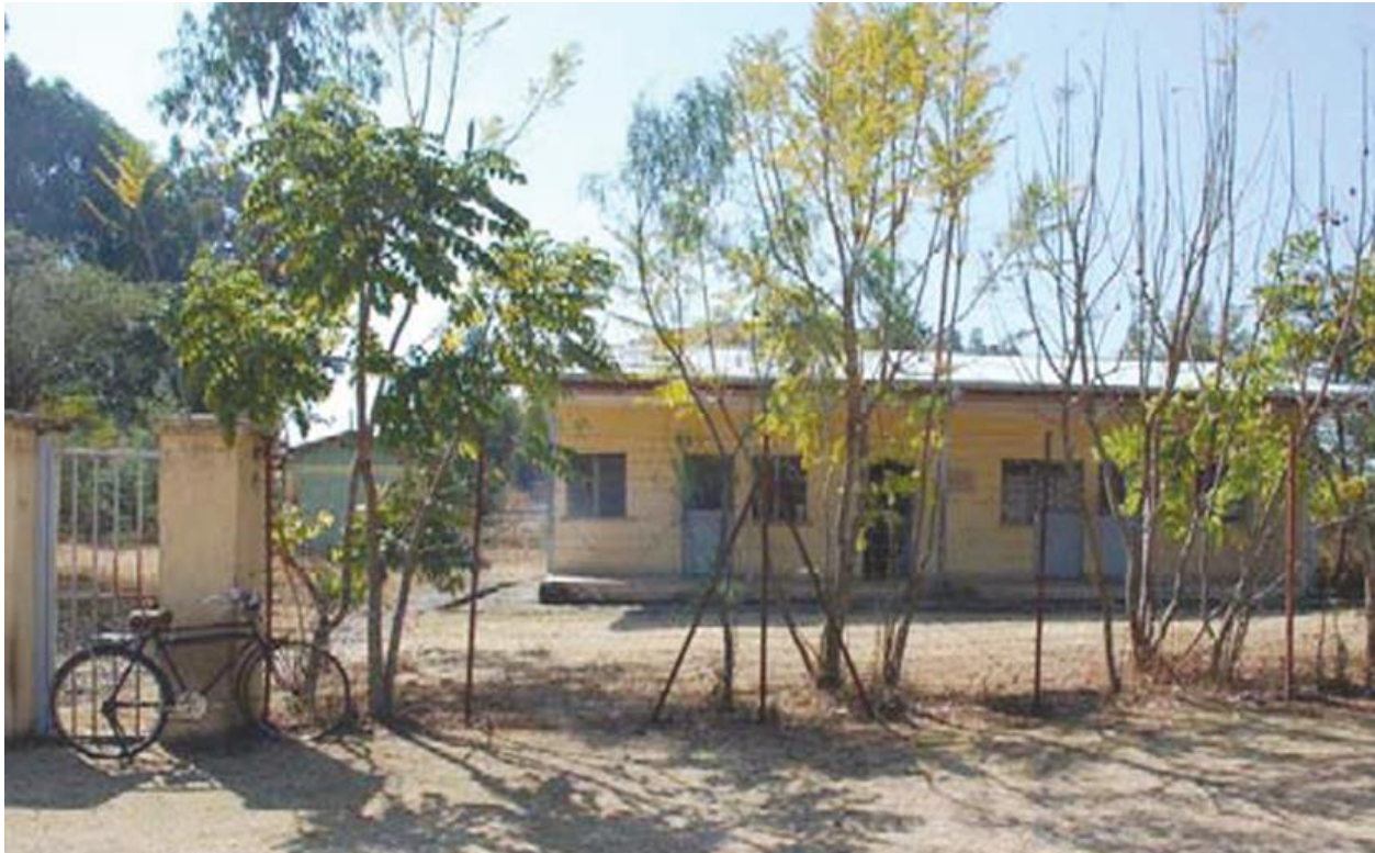
Figure 1.3 More than 14,000 Health Posts have been constructed as part of the HSEP program.(Photo: Ali Wyllie)
